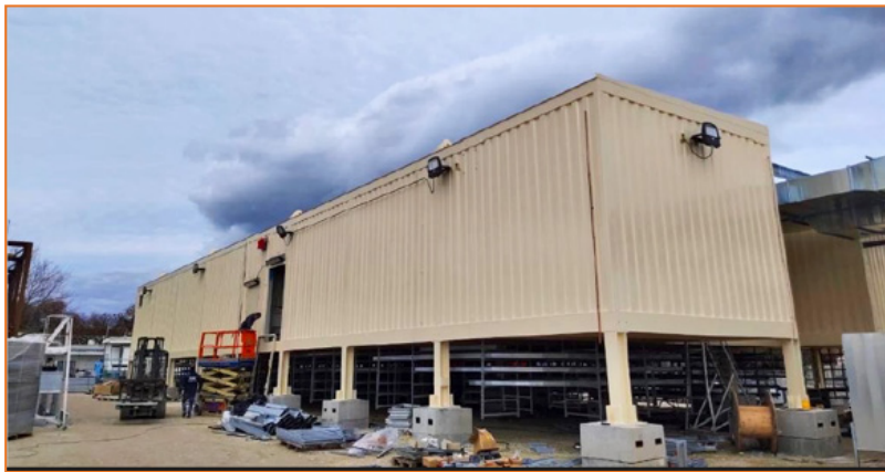
Prefabricated assembled E-houses to be used onsite.
